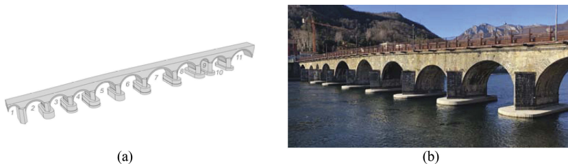
Figure 7. Azzone Visconti bridge: a) model representing the current shape (adapted from di Prisco et al. 2019) and b) current view.
