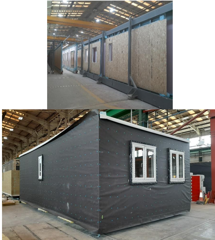
Fig. 1. Production line of CFS wall system for modular applications. © 2021.
