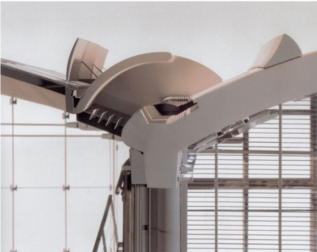
Fig. 4. Ingenhoven Overdiek und Partner , Lufthansa Aviation Centre , Frankfurt Airport, Frankfurt (© Courtesy of Ingenhoven Overdiek und Partner ).
