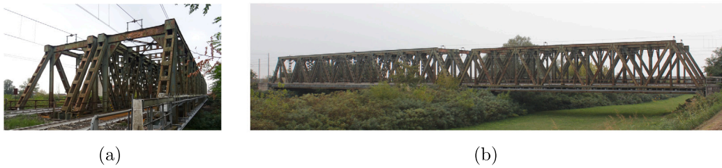
Fig. 1. Warren truss bridge under analysis. (a) Frontal view. (b) Side view.
