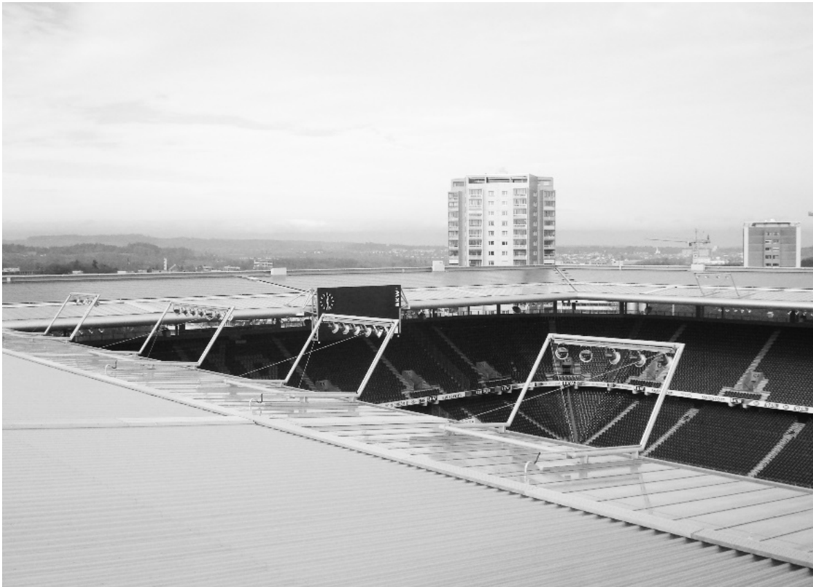
Figure 9. Wankdorf Stadium (Stade de Suisse, Bern, 2005). An urban stadium that until recently was the largest roof-mounted photovoltaic power plant in Europe, it houses public functions such as university spaces.
