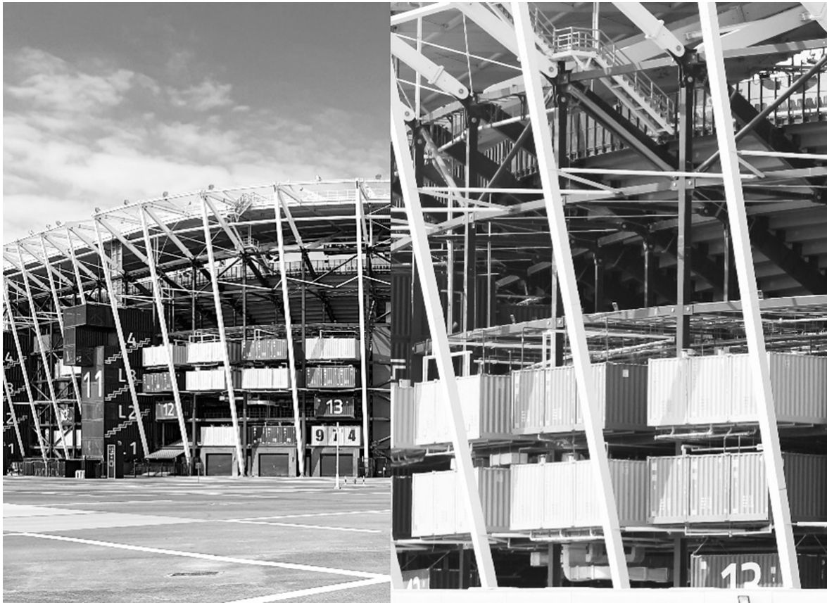
Figure 11. 974-Stadium (Doha, 2021), is the first example of a stadium that can be completely demountable. Built with recycled containers for the Qatar World Cup, it is the symbol of a quite consolidated technological trend for large sporting events to build infrastructures that are partly or completely adaptable, demountable, flexible and resilient (the latest Olympics in Paris are a clear example of this approach).
