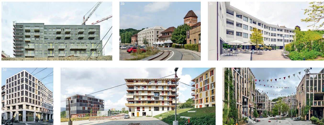
3a BHSF Architects, Warmbächli Cooperativa - Holligerhof Güterstrasse 8, Berna (2015-2021) 3b Baumschlager Eberle, 2226 Emmenweid, Emmenbrücke (2018) 3c Graber Pulver, Alterszentrum, Erlenbach (2016-2018) 3d Sergison Bates, Rue du Cendrier, Ginevra (2011) 3e LBL Architectes, Ecoquartier Meyrin Vergers - Cooperative Polygones Bonhôte Zapata - Coop. Equilibre, Ginevra (2015-2018) 3f GWJ Architekten, Huebergass, Berna (2019-2021) Foto Stefano Guidarini
