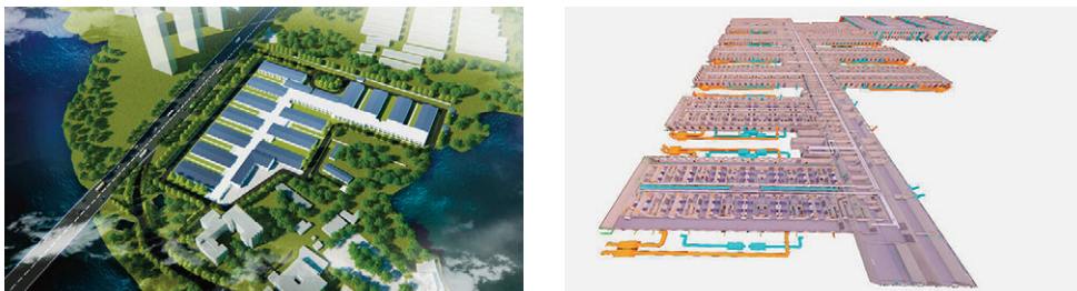
Fig. 8, 9 | Wuhan Huoshenshan Hospital is the world's first large-scale temporary facility built in record time to accommodate people infected with Covid-19. Designed in 24 hours with BIM methodology and created by CITIC Architectural Design Institute and China Construction Third Engineering Bureau, by a team of approximately one thousand five hundred workers and five hundred construction machines, at the request of the Wuhan municipal construction unit (source: redshift.autodesk.it; credit: CITIC ADI).
