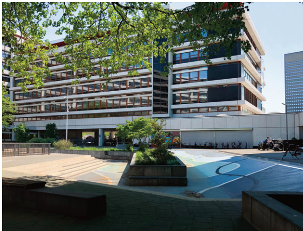
Fig. 13 | Watersquare in Rotterdam by De Urbanisten (credit: L. Errante, 2018).
