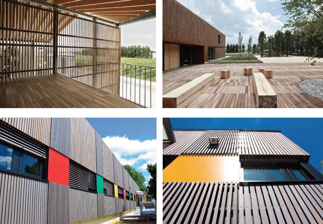
Fig. 1 | Pizzolato Winery in Villorba (Italy), designed by Made Associati (2013-2016). In this project, the use of beech wood for the building's cladding and external flooring was experimented with in an ecological way. This is PEFC-certified wood from the nearby Cansiglio beech forests. The wood was left natural for the floors and furniture (about 1,500 square metres), while for the exterior cladding it underwent a thermo-baking treatment that makes it more resistant to atmospheric agents, without precluding its recycling at the end of its life (credit: madeassociati.it, 2019).
