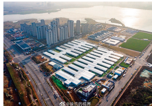
Fig. 11 | Global view of off-site modular units in the Wuhan Leishenshan Hospital project (source: archdaily.com).
