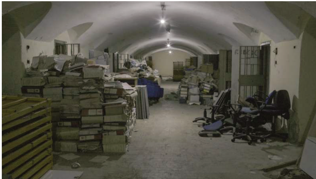
Figure 5. The ReverseLab space in San Vittore before the regeneration works
