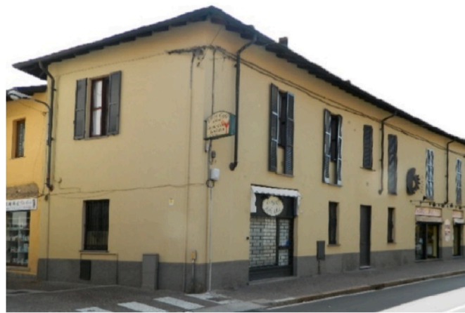
Fig. 9. Town of Desio (MB): recurrent masonry building typology in Lombard urban context of the beginning of 20th century (in CARTIS database named MUR1 in the historic centre named CO1).
