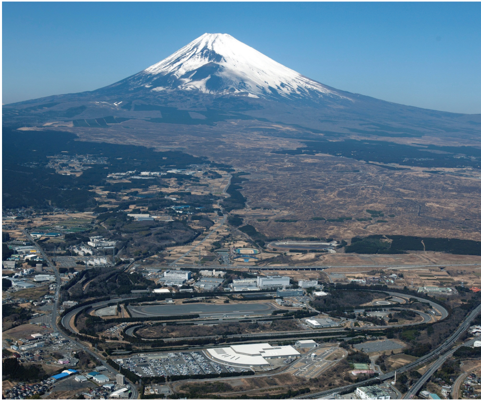
Figure 5. The site of Woven city before starting the construction works. (Source: Toyota Woven City. https://global.toyota/en/download/14221319/ )
