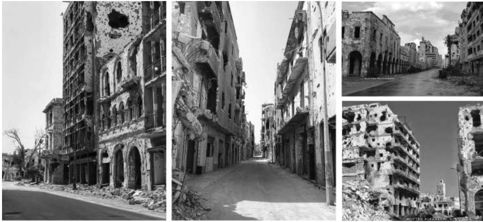
Figure 3. Damage to the Old City center buildings. (Left and middle photos by Bulifa, 2022. Photos on the right by Muftah Al Khashmi, 2021)
