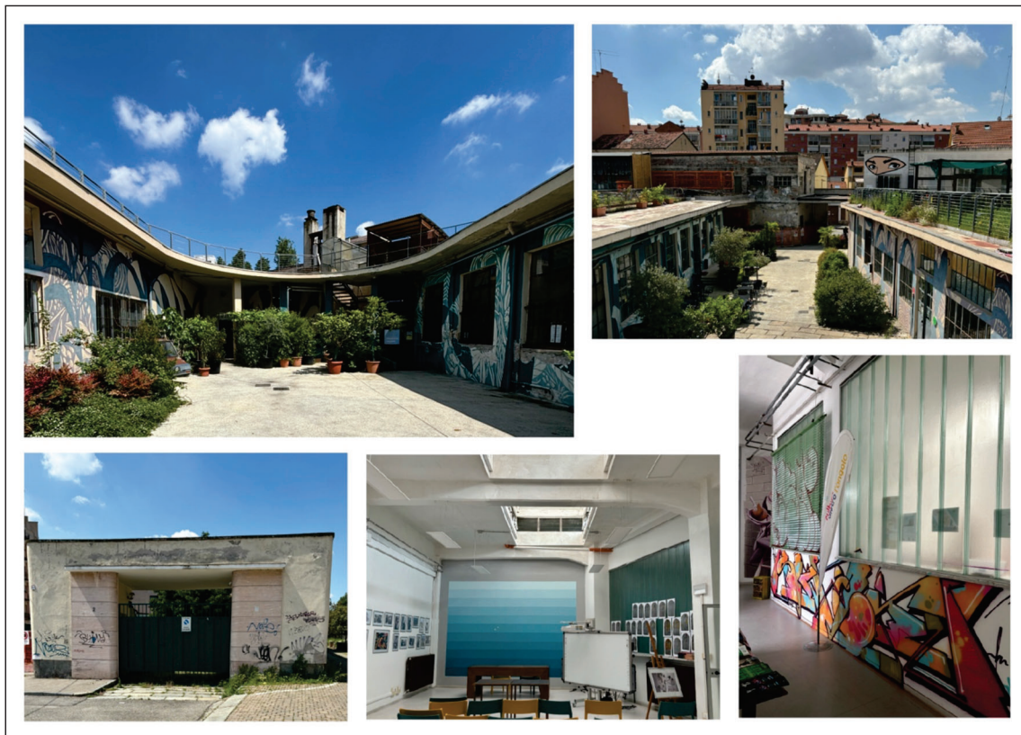
Figure 2. Beeozanam in current days: courtyard, largo Giachino entrance and interiors (pictures by the authors) .
