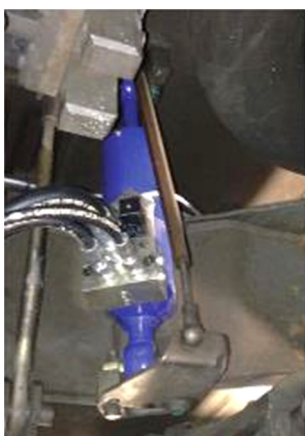
Fig. 19 Actuator replacement in Regina 250 [36, 37]
