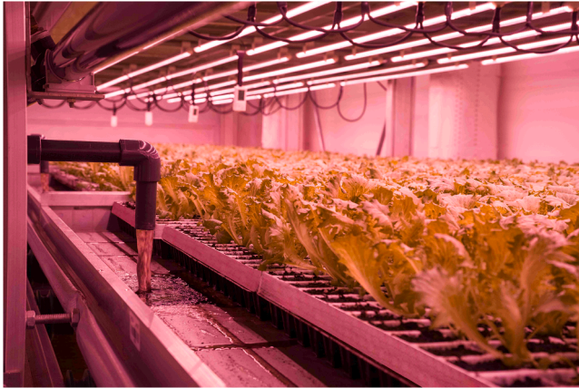
Fig. 2. Ebb and Flow irrigation system at Agricola Moderna.
