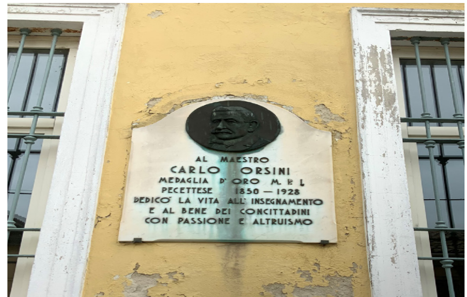
Detail of the facade of the school building.
