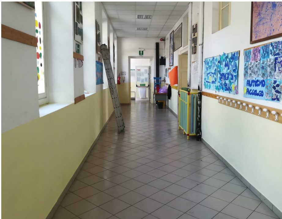
Corridor at the ground floor in 2021.
