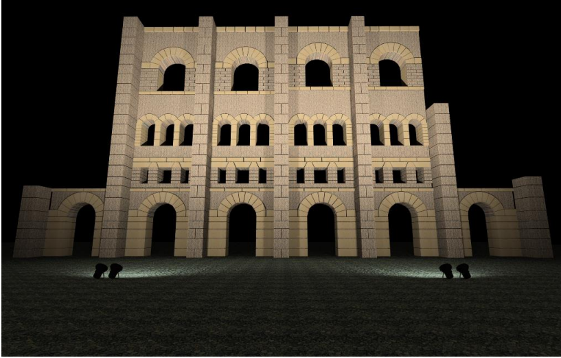
Figure 4.40 Artificial lighting of the façade of the Roman Theater in Aosta, 20 m high and 28 m wide at the base, by means of two pairs of floodlights located on the ground 12 m away from the building.
