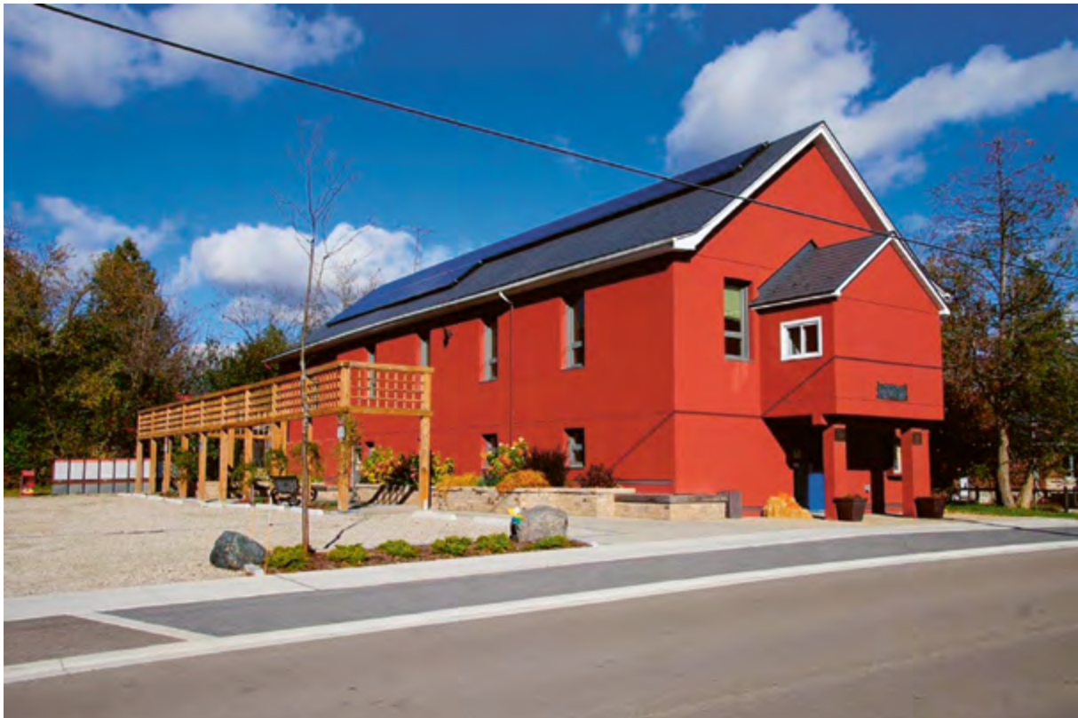
Figure 1.1.5. Eden Mills Heritage Hall after the deep thermal energy retrofit and photovoltaic installation. (Credit: Sword, 2010).
