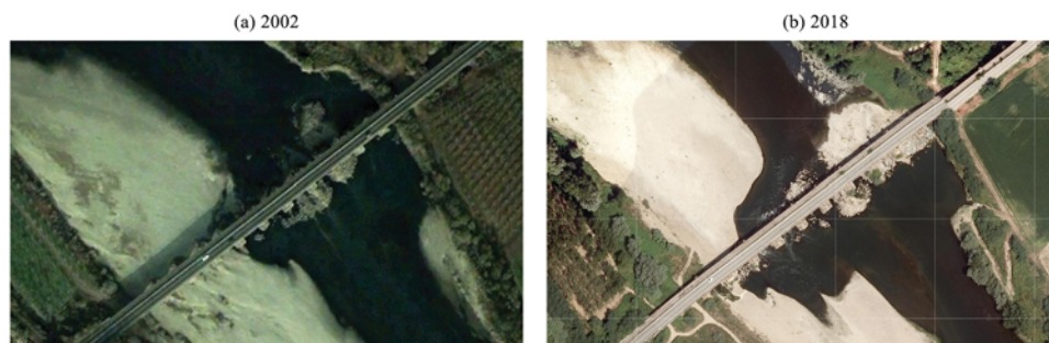
Fig. 3. Satellite images of the Sesia River (flow direction from top-left to bottom-right): before (a) and after (b) the rock armour installation around the piers of the left side channel.
