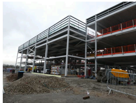
(ii) Outside view of the building (Dining/main hall and teaching block)
