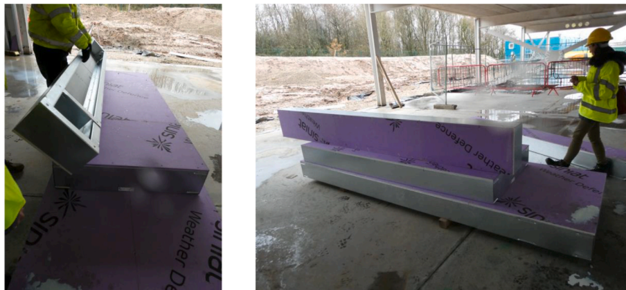
Fig. 3. Pre-assembled lightweight exterior infill wall panels.
