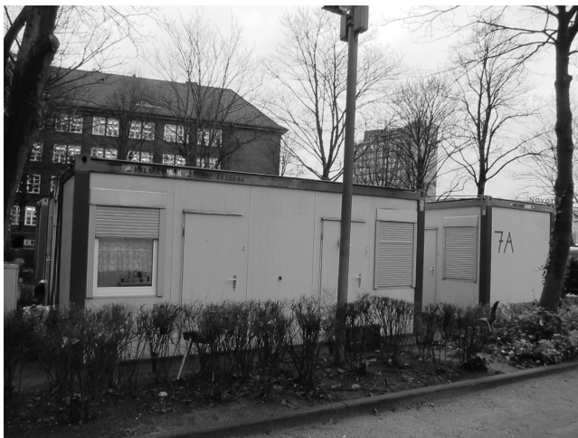
FIGURE 21.2 Containers as part of the Winternotprogramm Hamburg.
