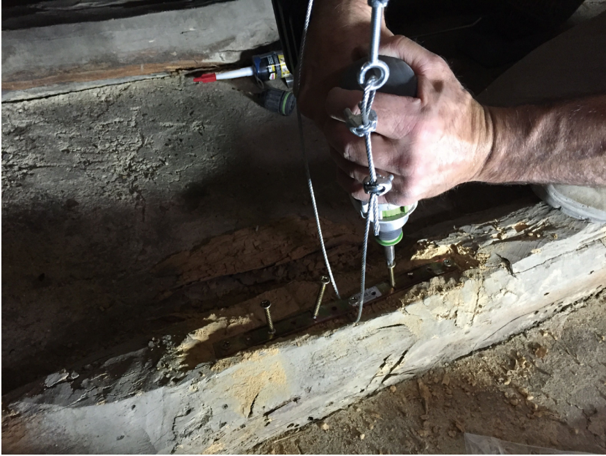
FIGURE 21 Fixing phase of the iron plaque with wood screws
