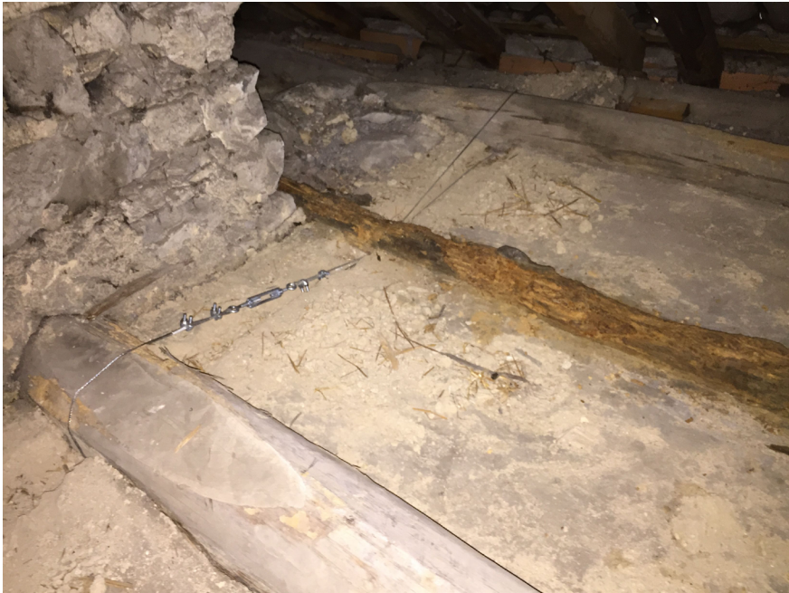
FIGURE 16 Execution phase described in Fig. 15
