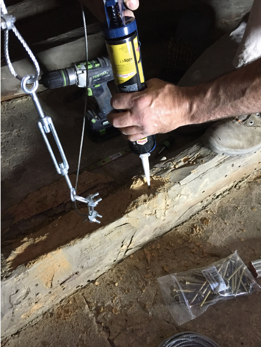
FIGURE 20 Injection of adhesive inside the pilot holes
