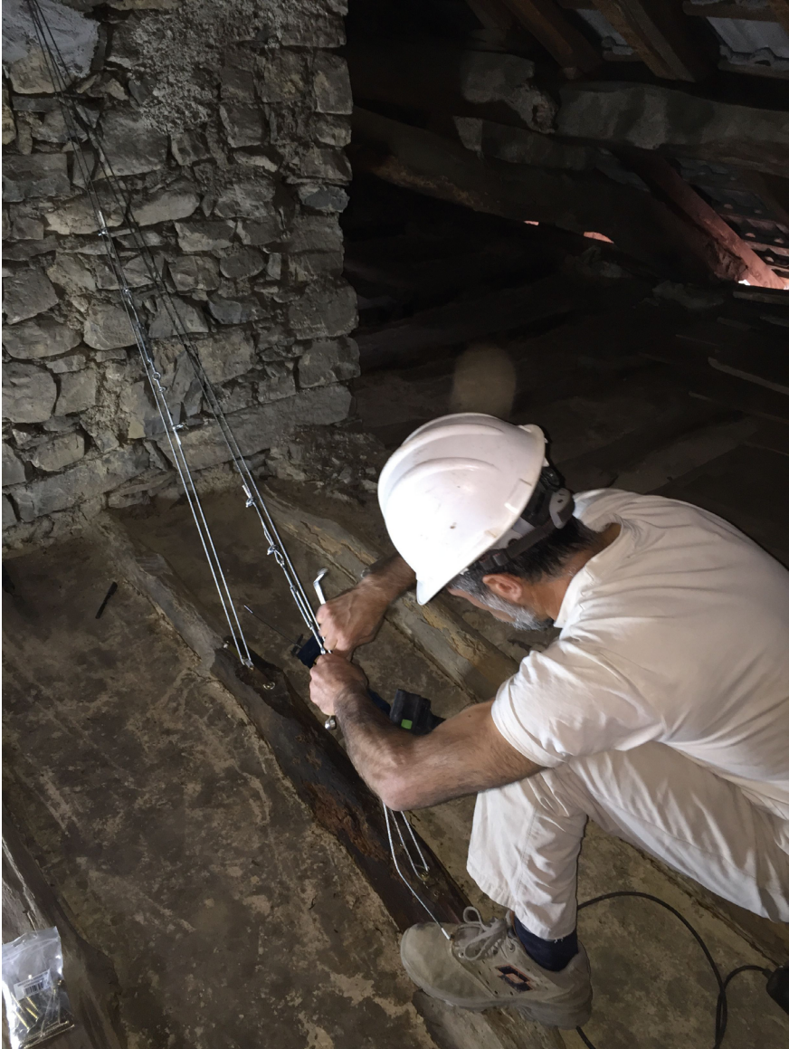
FIGURE 14 Execution phase described in Fig. 13
