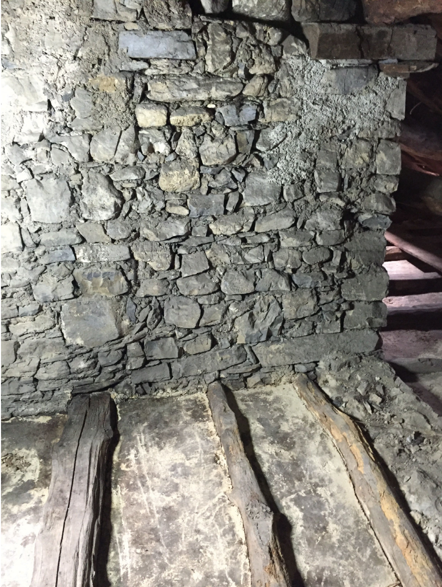
FIGURE 7 Extreme variability of spacing, processing, and diameter of timbers
