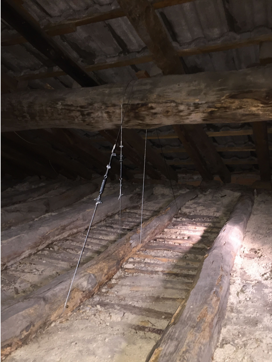
FIGURE 18 Execution phase described in Fig. 17
