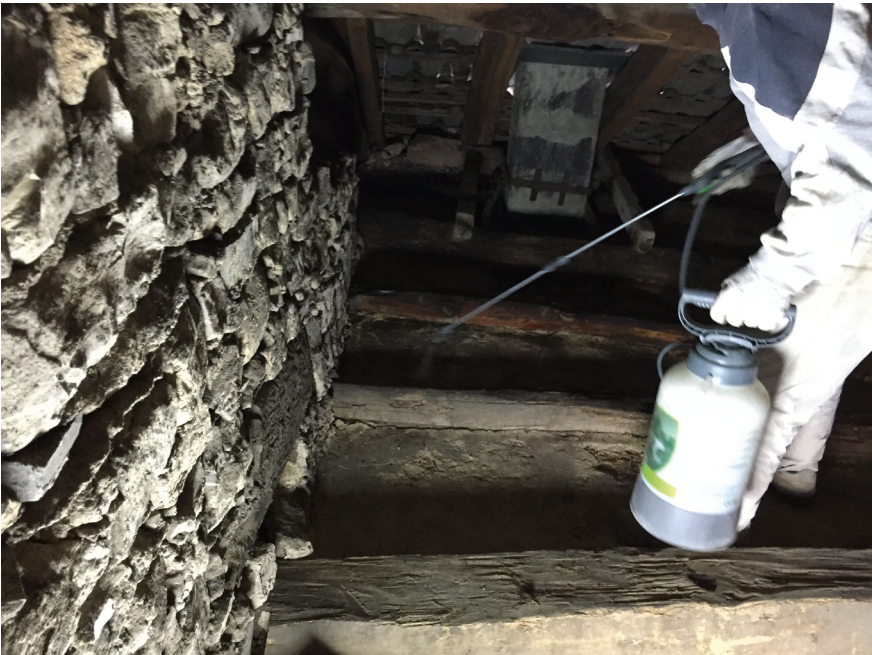
FIGURE 22 Spray treatment with a chemical preservative
