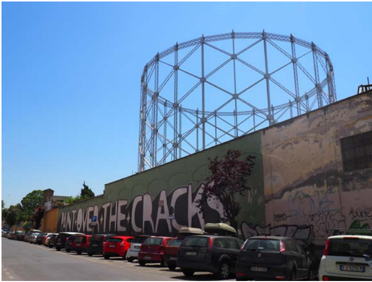
Fig. 2 The gas implant (Gazometro) is one of the main landmarks of the Ostiense area. Credits: Daniela D'Avanzo.
