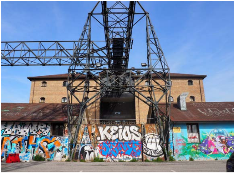
Fig. 4 The contrast among the materials used for the constructions alongside the graffiti painted highlight both the industrial and contemporary mood of the area. Credits: Daniela D'Avanzo.
