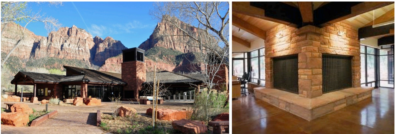
Fig. 3.8-4 – Zion National Park Visitor Center (left) and cooling tower outlet (right)
