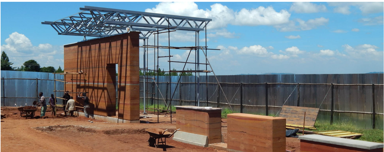
Construction stage © Emergency NGO
