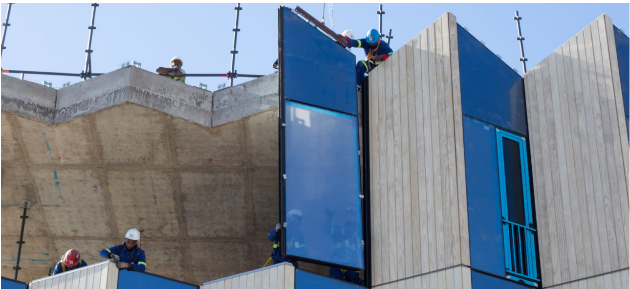
Construction site © Arup
