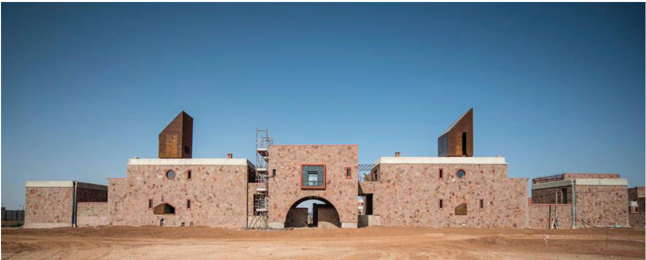
Construction site © Mohammed VI Polytechnic
