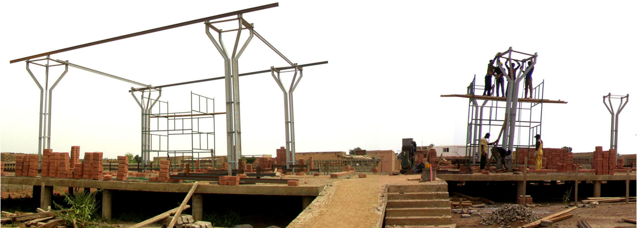
Construction site © FAREstudio
