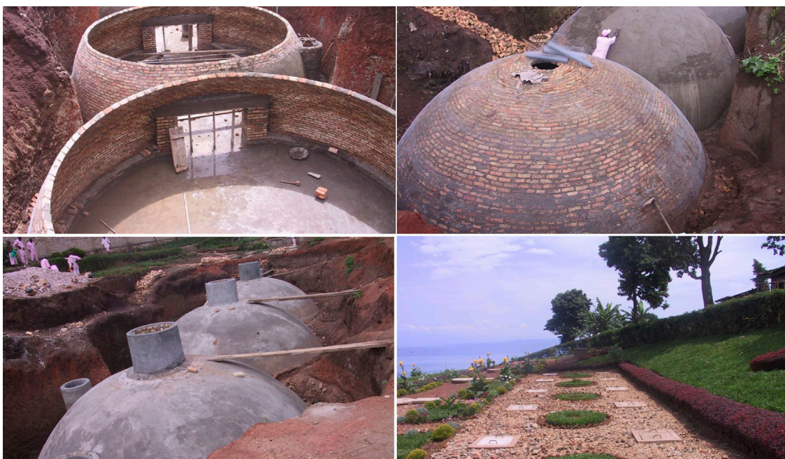
Fig. 5.2-5 – Digesters construction stages - Sources: G. P.Nembrini, A. Kimaro, Using Biogas Plants for Treatment of Urban Community Wastes to Supply Energy and Improve Sanitation , presented at the Expert Group Meeting on "Energy Access for the Urban Poor", December 2006, Nairobi
