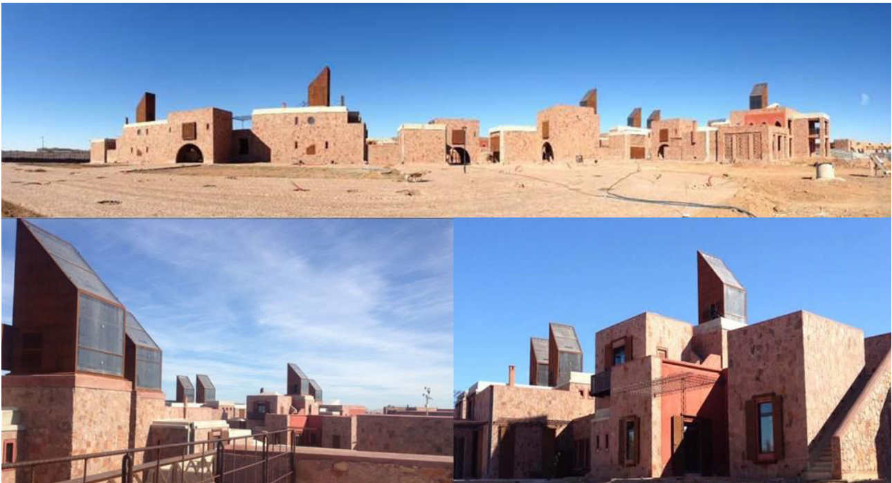
Construction site © Mohammed VI Polytechnic
