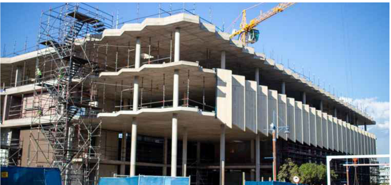
Construction site © Arup
