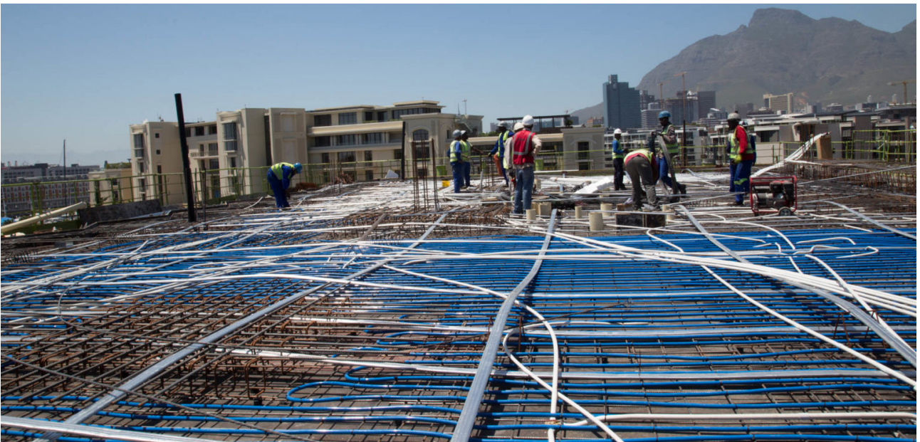
Construction site © Arup
