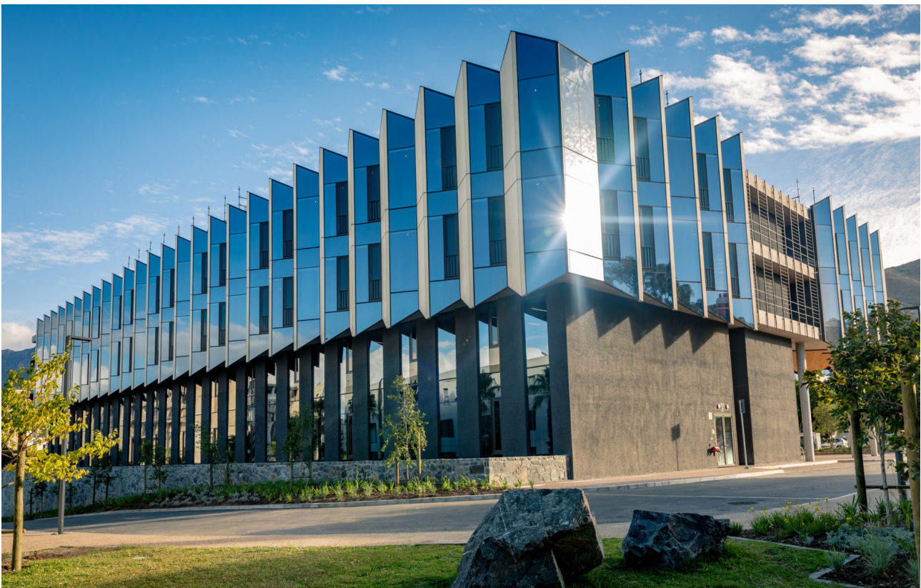
Exterior view © Arup
