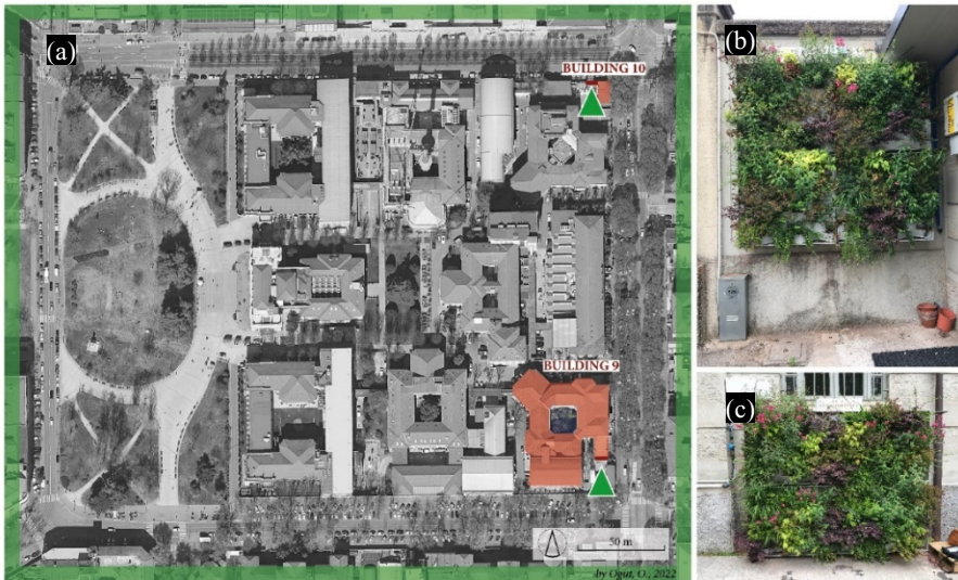
Fig. 1 (a) The VGS location in POLIMI campus: on the façades of building 9 and 10. (b) VGS on building 10. (c) VGS on building 9.
