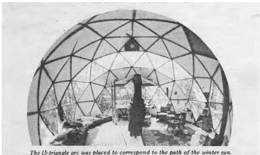
The 15-triangle arc was placed to correspond to the path of the winter sun.
