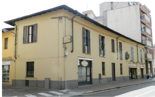
Fig. 6. Recurrent masonry building typology named MUR1 in the historic center of Desio (MB).
