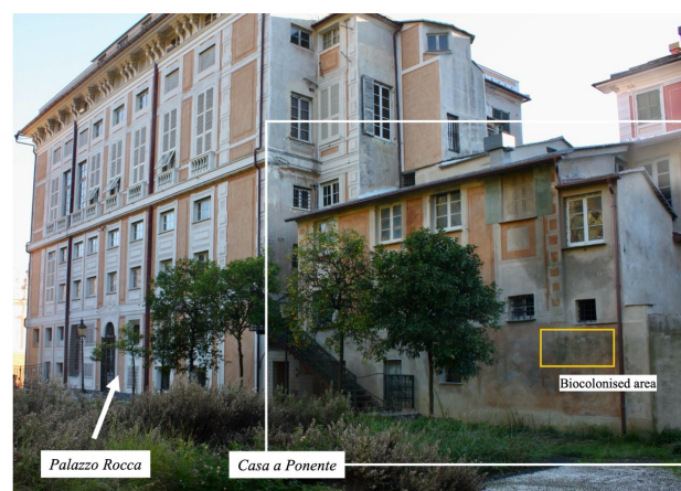
Figure 1. General view of Palazzo Rocca and the Casa a Ponente (white square), Chiavari (Italy). The yellow frame indicates the pilot area experiencing recolonization and is selected for the biocidal treatment applications and LCA evaluation.
