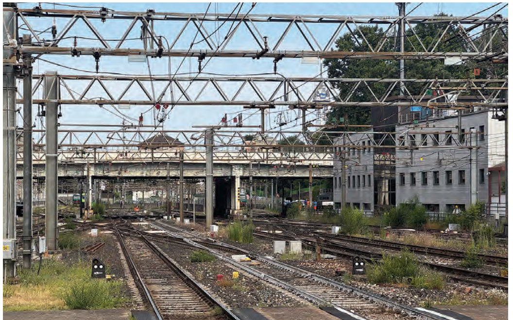
Fig. 8 | Milano Cadorna station and adjacent station building: current state (credit: M. P. Vettori, 2026).
