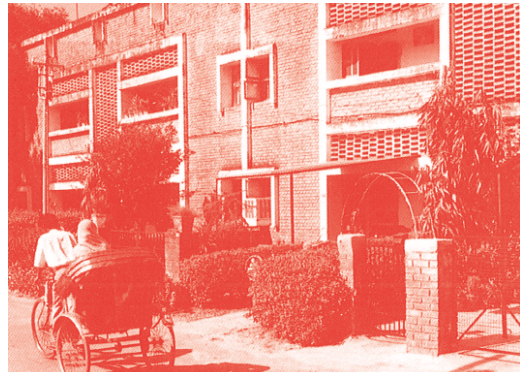
View of the Door step / Verandah
