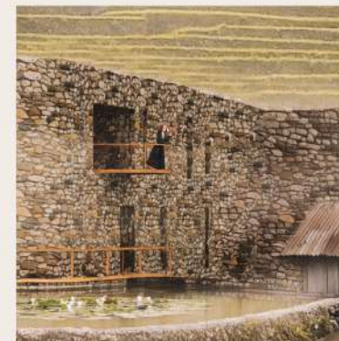
B. viewing decks overlooking the rice terraces
