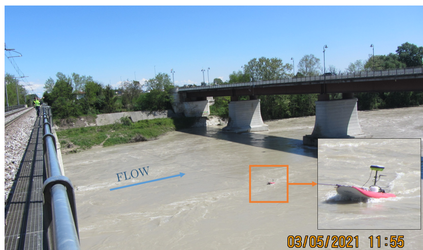
Figure 5. Photograph captured during the May 2021 measurement campaign from the Piave railway bridge. The image shows the ADCP mounted on a vessel, controlled by a rope from the bridge. To position the vessel onto the water surface, it is carefully lowered to the water's surface using a rope. Once situated in the water, it is slowly maneuvered from one bank to the opposite one.
