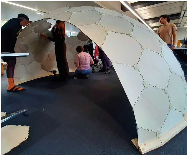
Fig. 2. The ECHO shell during construction. The panels require some external support during assembly, to counteract bending moments; however, support can be removed after assembly.
