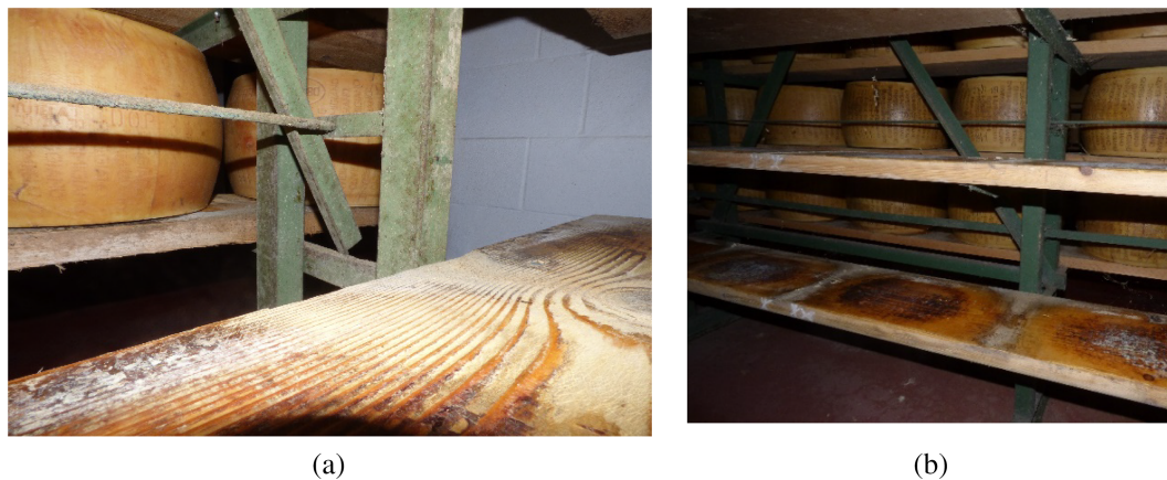
FIGURE 5 Typical vertical bracing systems for (a) type CR1 and (b) CR2 type
