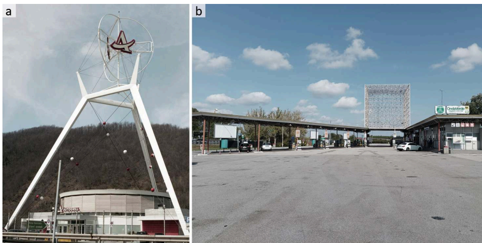
The autogrill by Angelo Bianchetti in Ronco Scrivia, 2018 (a) and the petrol station by Costantino Dardi in Mestre (Italy), 2021 (b).
