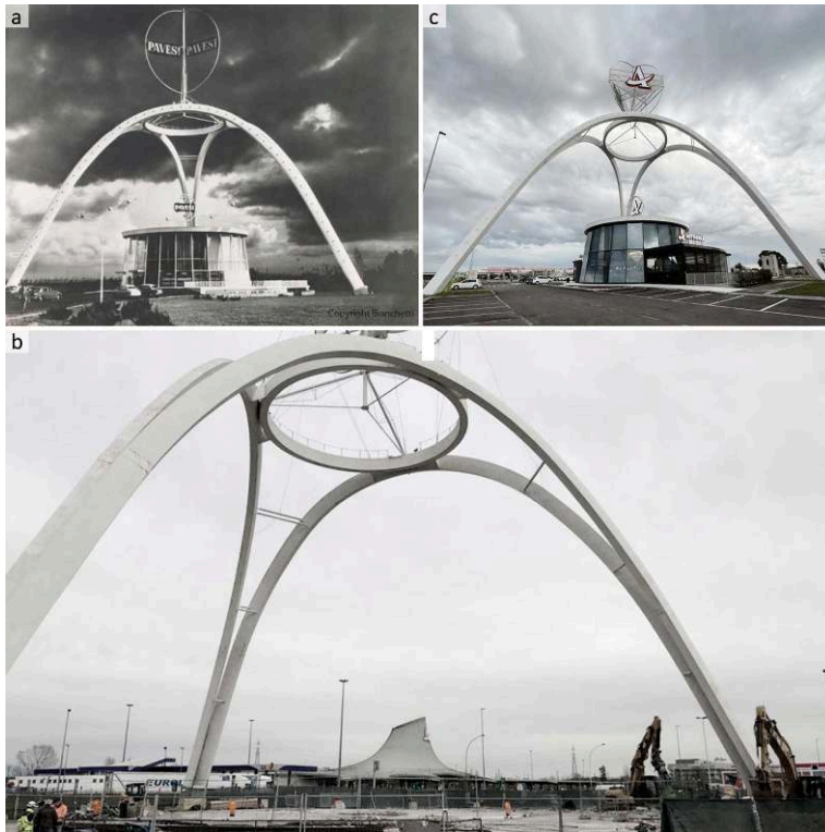
Autogrill by Angelo Bianchetti in Lainate, Italy, in the 1960s, photo from J.J. Bianchetti Archive / Como (a), after the demolition in 2020, photo taken from https://bit.ly/3l2hmav (b), and current state (2021) (c). The steel overhead structure has been preserved.
