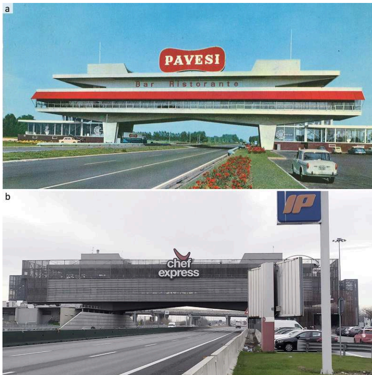
Autogrill by Angelo Bianchetti in Novara, Italy, in the 1960s, Pavesi postcard from J.J. Bianchetti Archive / Como (a) and in 2020, after the refurbishment by Massimo Iosa Ghini (b). The new shell hides the original concrete structure.
