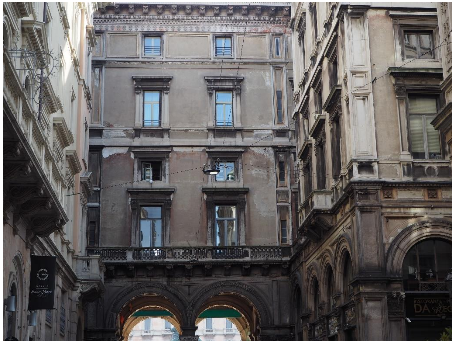
Figure 22 - Blackening and decay on historical buildings in the centre of Milan.
