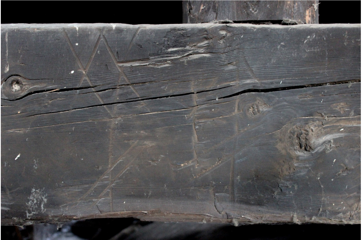
Fig. 11. Trading mark on the west side of the tie-beam of the T7 truss. (Photo by Emanuele Zamperini).
