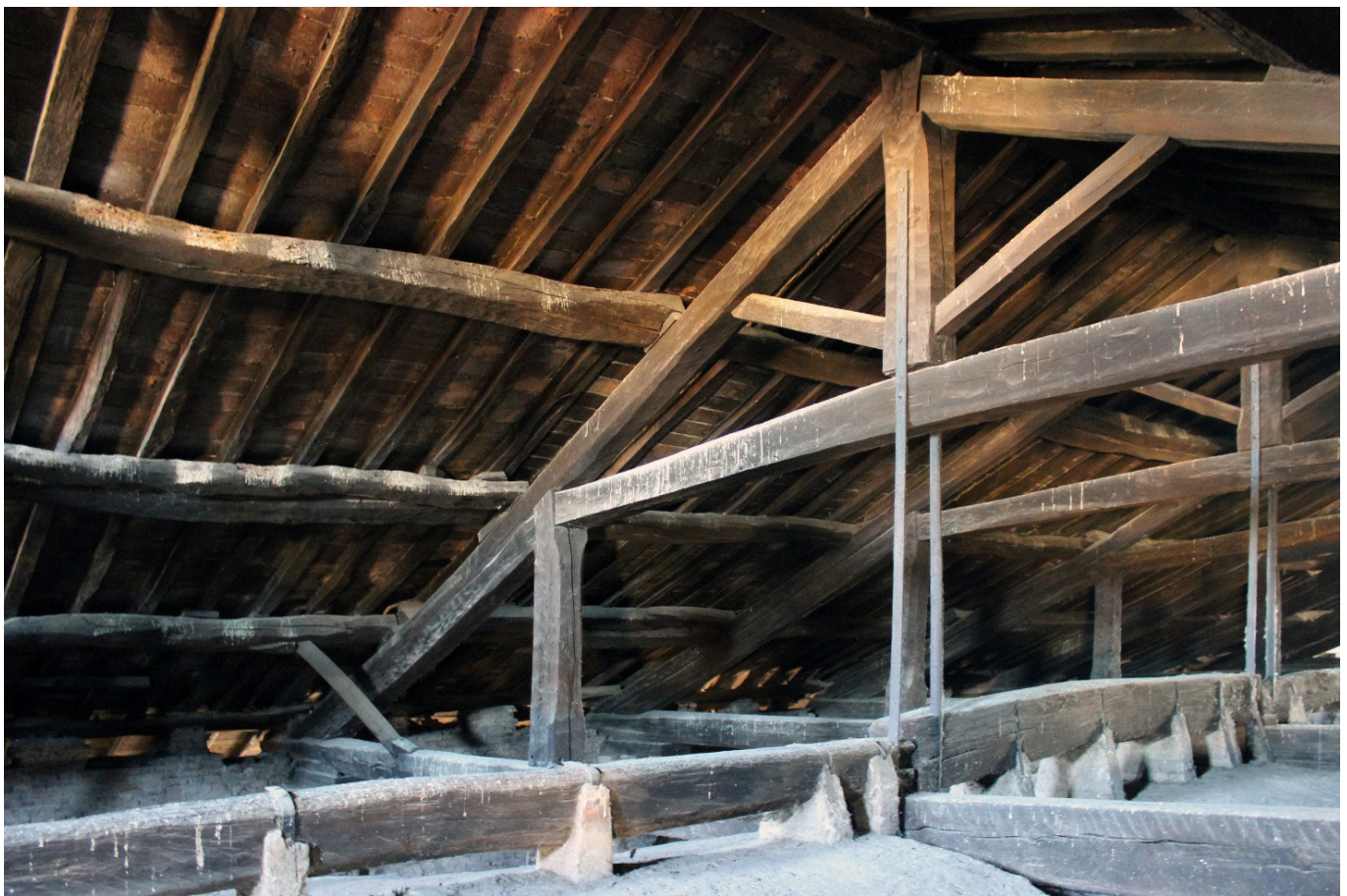
Fig. 6. Unmodified truss of the first phase: T3 truss seen from the north-east. (Photo by Emanuele Zamperini).
