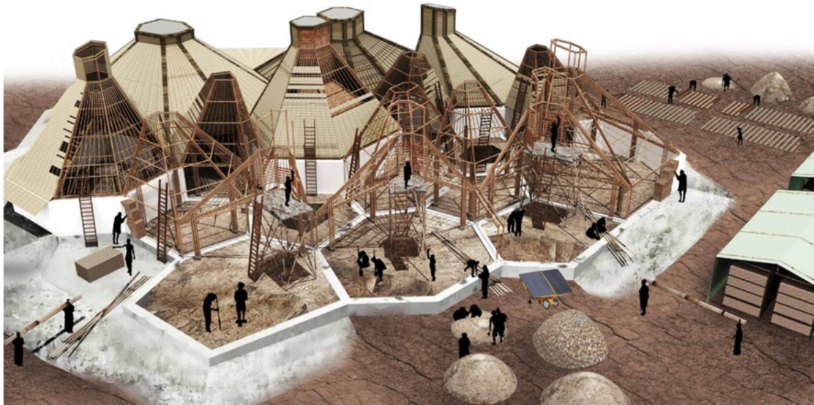
Figure 21. Low-tech construction logic of the school prototype, including earth-based wall construction, bamboo structure, and on-site execution.
