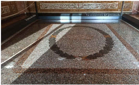
Figure 3. The Sala degli Arazzi and its floor. This picture puts in evidence some obstacles for the survey: the presence of strong light from the window, the reflection of the pavement together with the obstacles present in the room and the decay of the floor
