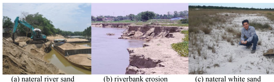
Fig. 1 River sand mining causes landslides and gradual loss of agricultural land
