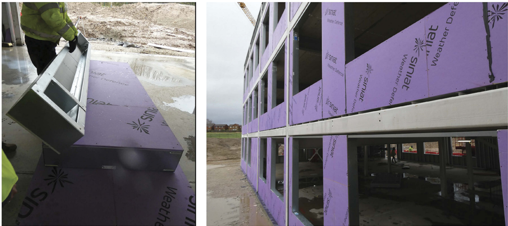
Figure 3. Prefabricated panelised infill wall with exterior plasterboard (photos taken by the authors on December 2021 in the Greater Manchester area, UK).
