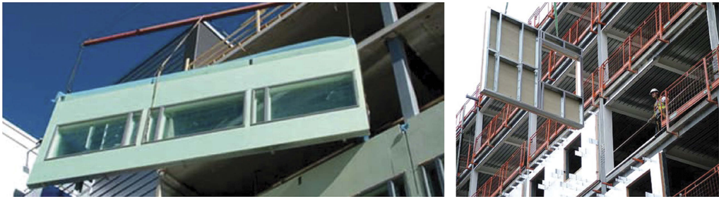
Figure 2. Installation of lightweight infill wall in a primary structural frame (images from SCI, 2008), (left): Prefabricated infill wall with cladding, windows, and light steel frame, and (right) prefabricated infill wall with exterior plasterboard, windows, and light steel frame.
