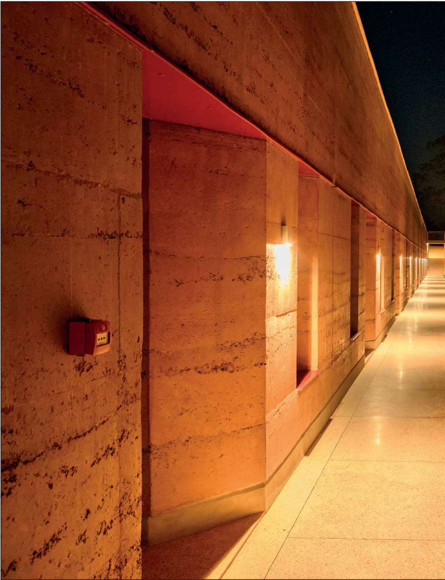
Emergency NGO Onlus, Renzo Piano Building Workshop, TAMassociati, Childrens Surgical Hospital , Entebbe, Uganda, 2013-2020, © Emmanuel Museruka. A detail of the walls made in rammed earth.
