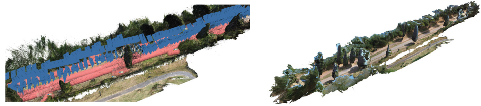
Figure 18. (left) the final Dense Cloud product is achieved by aligning and merging the post-processed Dense Cloud of the 360° images (in pink, the 360° frames) and the cleaned Drone Dense Cloud (in blue, the drone frames). (right): the two chunks are aligned with Point Cloud assets settings and then merged to create a unified representation of the surveyed area.
