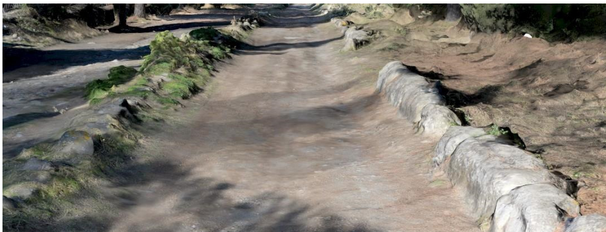
Figure 10. One of the first miles, where the Basolatium paved surface is not present, while Crepidines are visible.
