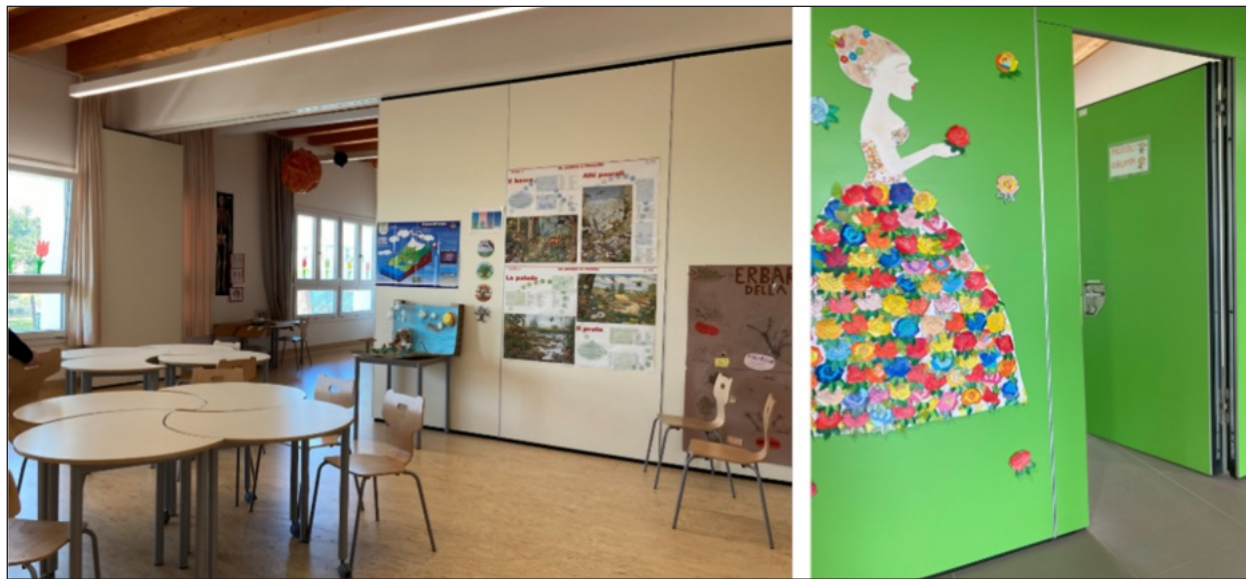
Figure 3. Foldable walls in laboratory spaces (left) and along corridors (right)).
