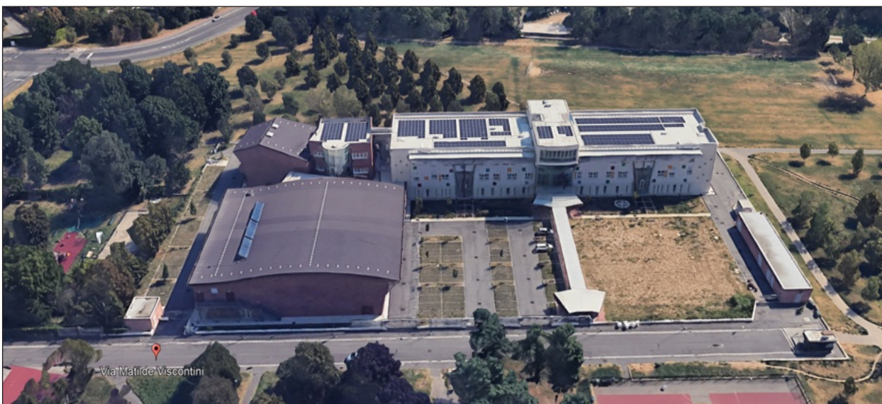
Figure 2. View of the school complex on Via Viscontini, Milan.
