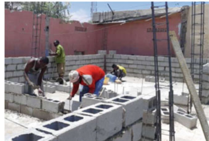
Walls are built with hollow concrete blocks and cement mortar.
