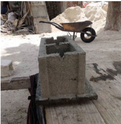
Concrete blocks are transported over the pieces of flat wood.
