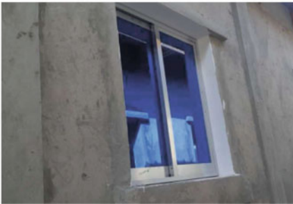
Single glass metal windows are installed.
