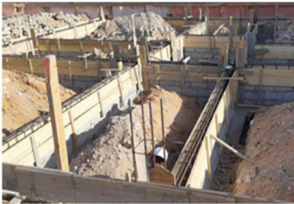
Wooden formwork are installed for bond beam works.
