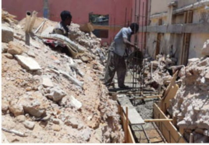
Concrete is placed and cured for foundation beam.
