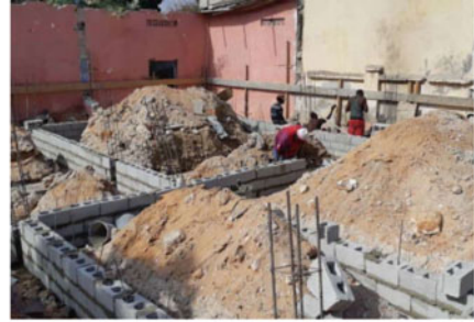
Layers of concrete blocks are placed for foundation beam construction.
