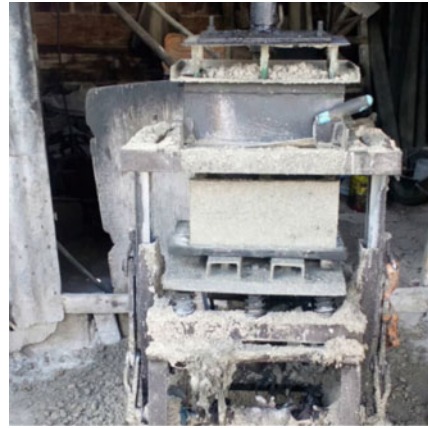
Concrete is manually compressed using compressing machine.
