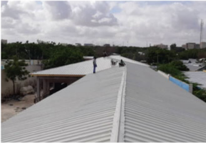
Galvanized corrugated iron sheets are placed as roof finishing.
