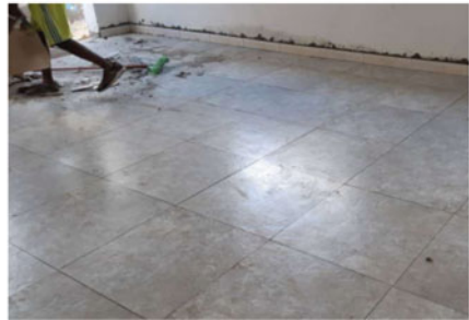
Ceramic tiles are installed as floor finishing.
