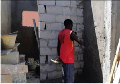
Cement mortar is applied as interior wall plastering.
