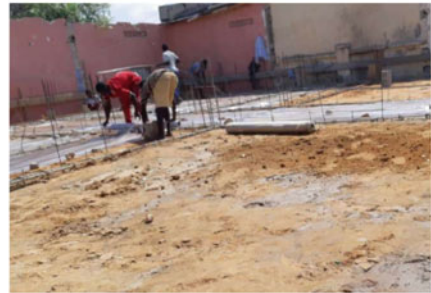
Waterproof membranes are lay down for covering the soil.
