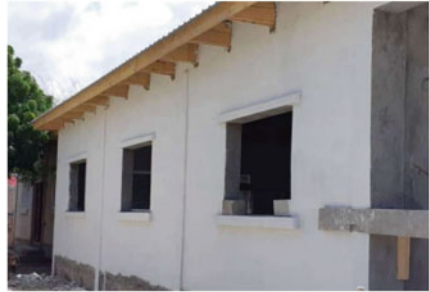
White plaster is applied both on exterior and interior walls.
