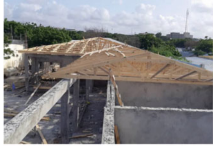
Wooden truss is installed for roof construction.
