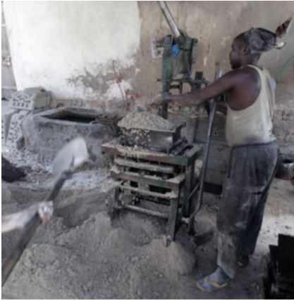
Concrete mix is poured into the brick cast.
