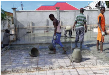
Concrete is gradually placed for floor slab.
