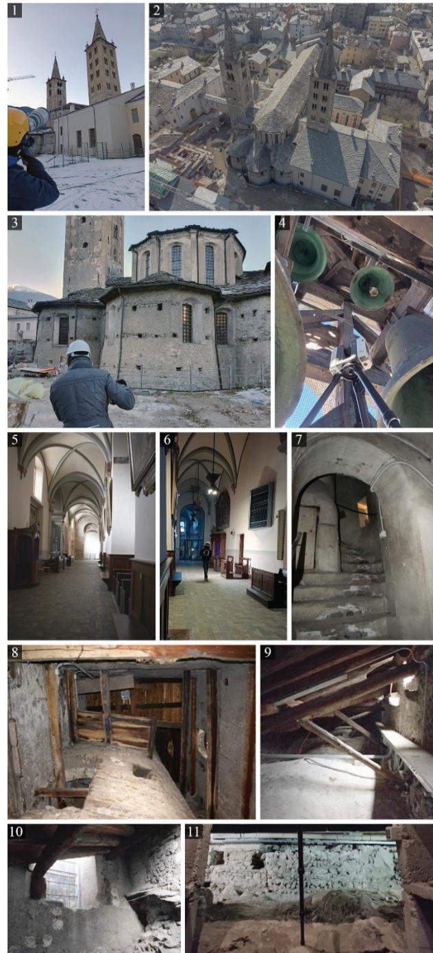
Figure 1. Images of the Aosta's Cathedral: exterior area of the apse (1, 2, 3), belfries (4), naves (5, 6), indoor view of the south tower (7, 8), attics (9, 10) and archaeological area (11).
