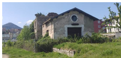
Figure 2. Pignola Station : photo from the on-site survey.
