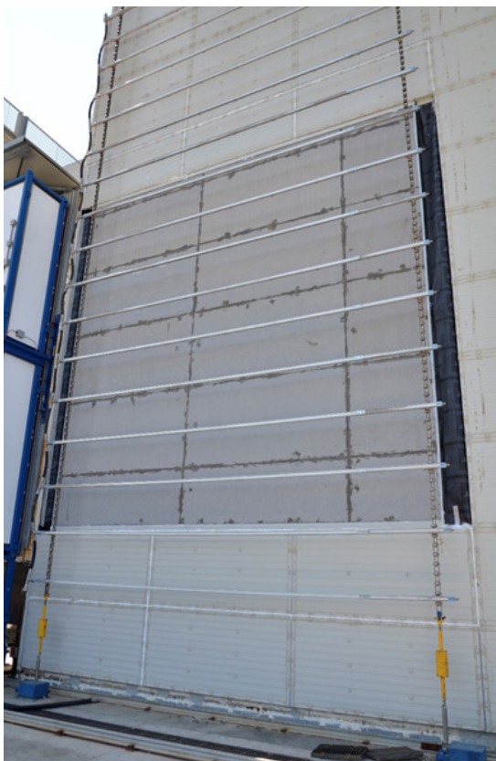
Fig. 30 - Campione sottoposto a prova nell'assetto sperimentale: Full Scale Mock-Up / Sample tested in the experimental setup: Full Scale Mock-Up (Source: Authors' elaboration).
