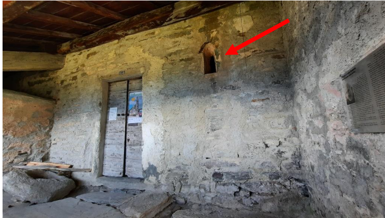
Figure 3: Location of the external probe (south-western wall, outside).
