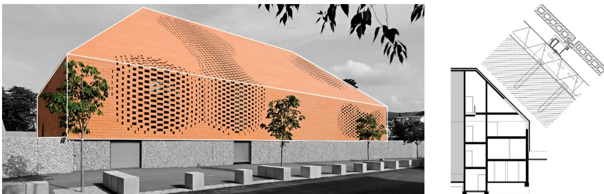
Figure 7. Terra-cotta cladding façade and detail - Pope John Paul II Hall by Randić & Turato
