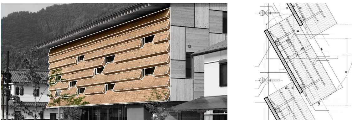
Figure 9. Straw units curtain wall and detail - Yusuhara Marche by Kengo Kuma & Associates
