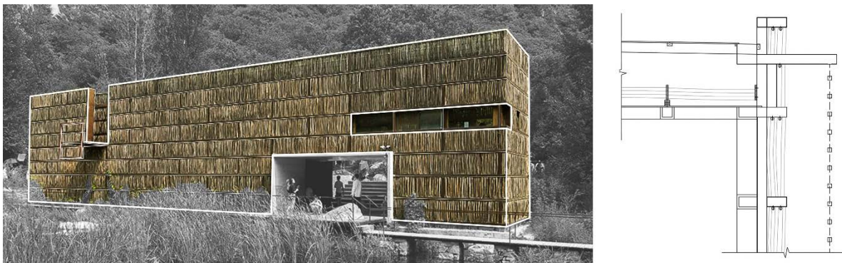
Figure 3. Wooden sticks façade and detail - LiYuan Library by Li Xiaodong Atelier
