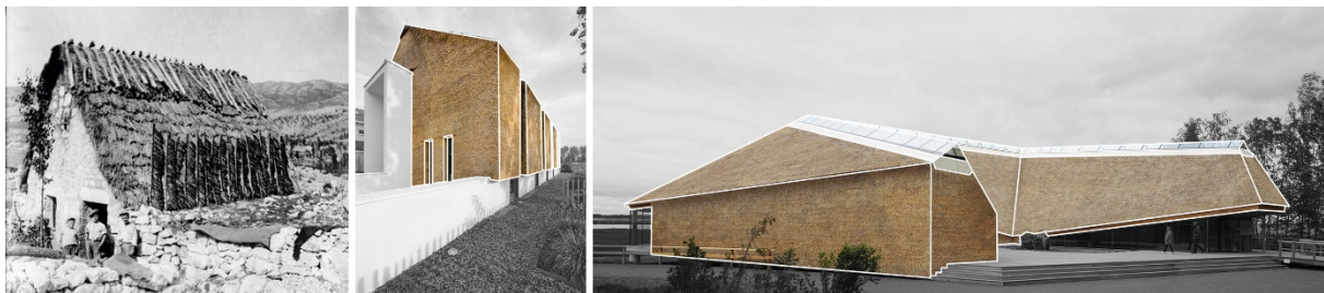
Figure 8. Straw as building envelope, from vernacular to contemporary - House in B&H, Posusje 1930; Living on the Edge House by Arjen Reas and Facts Tåkern Visitor Centre by Wingårdh AB
