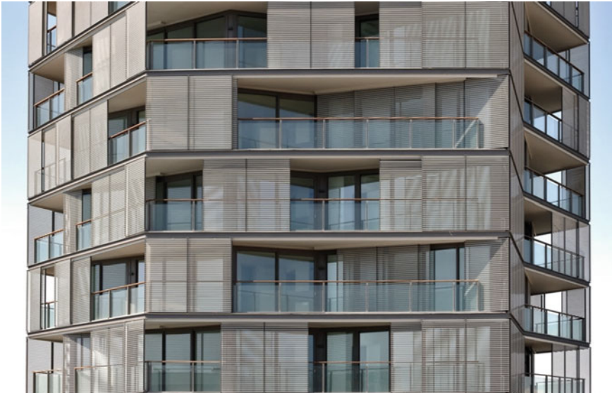
Fig. 1.17 Carlos Ferrater, Aquileia Tower , Jesolo. Interweaving the “intermediate spaces” beyond the curtain walls by suspending the façade structure from the roof: the surfaces are made up of a system of intersecting and sliding “sails”, capable of screening and defining the osmotic perception between inside and outside. © Courtesy of Schüco
