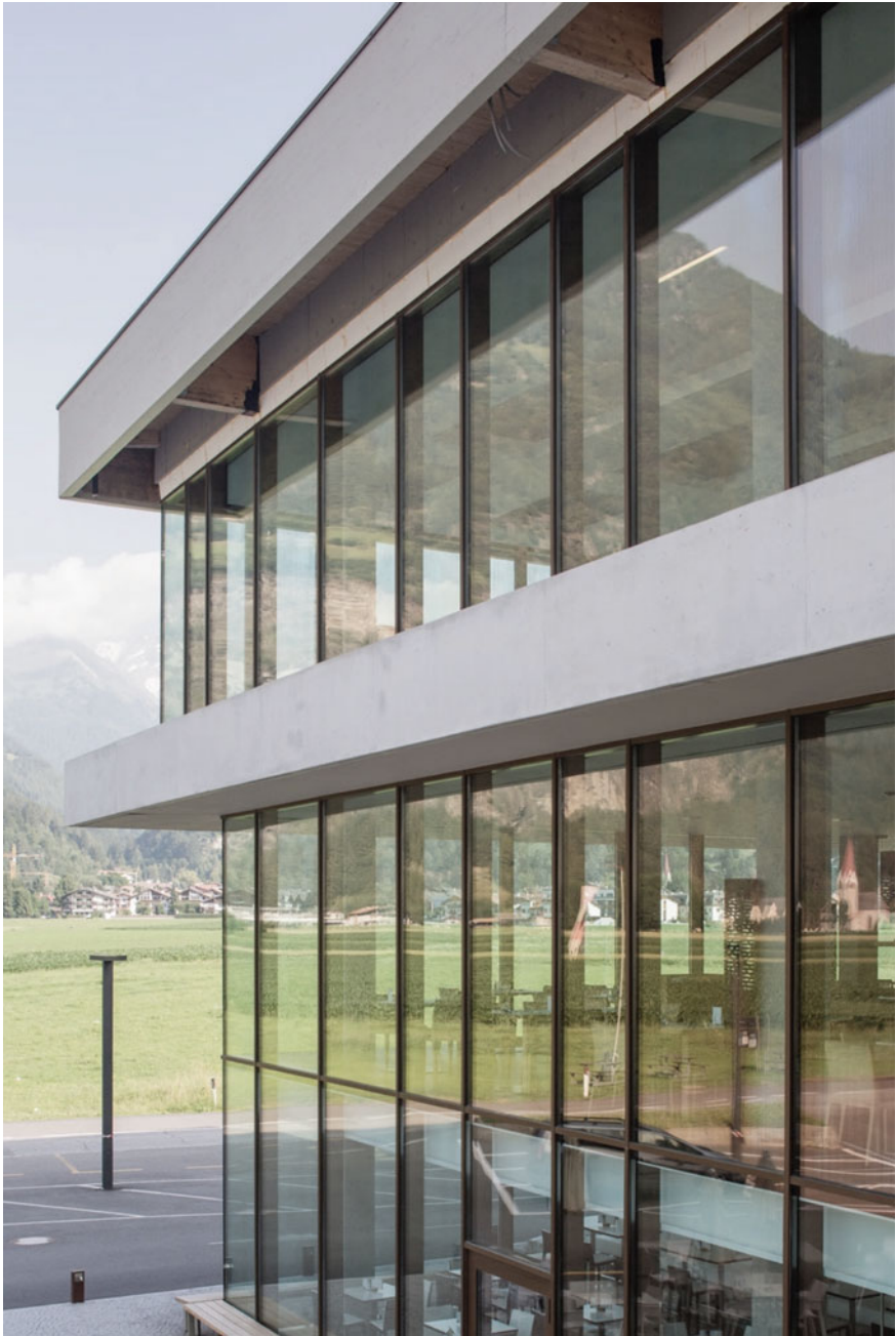
Fig. 1.1 Christoph Mayr Fingerle, Cascade Swimming Centre, Campo Tures (Bozen). Role of “transition” between internal and external spatiality of the envelope, understood as a modular apparatus warped from the load-bearing framework towards the glazed surfaces, inserted in the horizontal perspective composition. © Courtesy of Schüco
