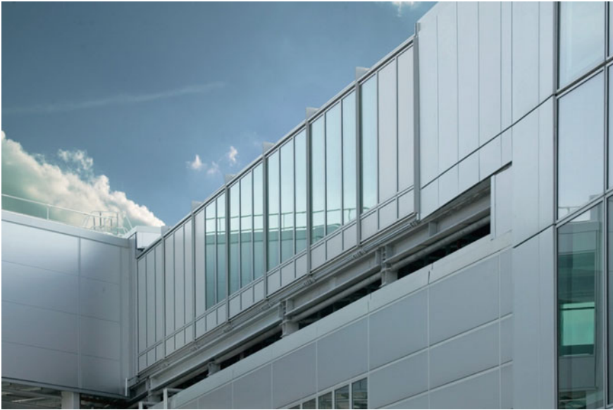
Fig. 1.3 Construction of pre-assembled modules. System designed according to the execution of serial units, which are mechanically assembled on the steel-framed decks and by means of the insertion of the upper enclosure on the open cells of the mullions. © Courtesy of Reynaers
