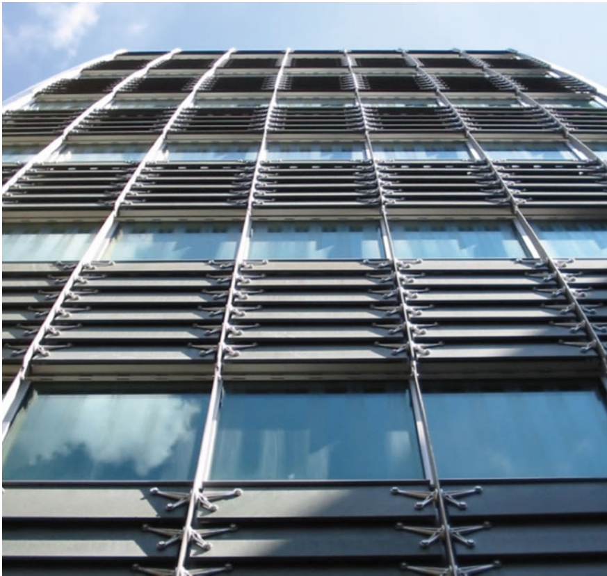
Fig. 1.12 Nicholas Grimshaw and Partners, Gresham Street Office Building , London. Use of transparent, osmotic enclosures, equipped with “hybridized” components and brought up to date with respect to the building tradition, within a modular grid: adoption of components and parts for the façades capable of bringing together the archetypal stylistic features of material culture and the canons of technical-productive innovation. © by the Authors
