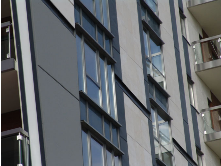
Fig. 1.4 Gergely Paulinyi and András Reith (Mérték Építészeti Stúdió), Prestige Tower , Budapest. Definition of the components according to the use of finished products, dimensionally coordinated and combined according to a homogeneous texture. © Courtesy of Mérték Építészeti Stúdió
