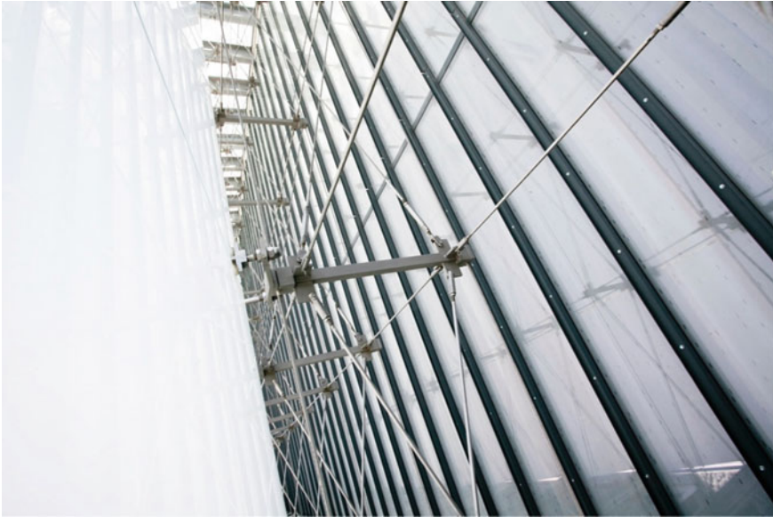
Fig. 4.20 Stelmach & Partners, CSK, Centrum Spotkania Kultur (“Centre for Encountering Cultures”), Lublin. Constitution of the section occupied by the tensile structure, within the space between the curtain walling and the structural glass modules. © Courtesy of Lilli Systems
