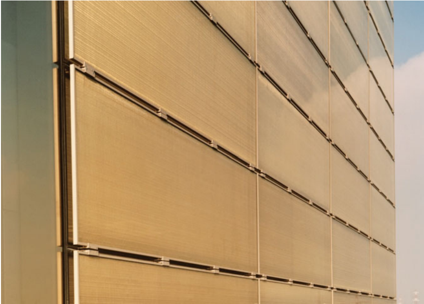
Fig. 1.10 5+1AA with Jean-Baptiste Pietri Architectes, Fiera Milano office building, Rho (Milan). Processes of “environmental interaction” of the envelope by means of technical solutions that “hybridize” serial typologies, through the aggregation of elements aimed at increasing the interruption of thermal transmission and interposing additional chamber sections. © Courtesy of Caviola
