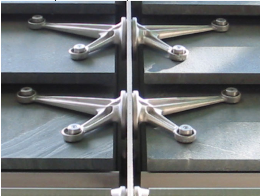
Fig. 1.13 Nicholas Grimshaw and Partners, Gresham Street Office Building , London. Physical and expressive hybridization between “natural” materials and prefabricated construction: envelope system determined by the cladding comprising the panels made from Broughton Moor’s green, flame-treated Cambrian slate stone slabs (Burlington production); the slabs are stacked according to horizontal development and are supported by the linear frame with point joints. © by the Authors
