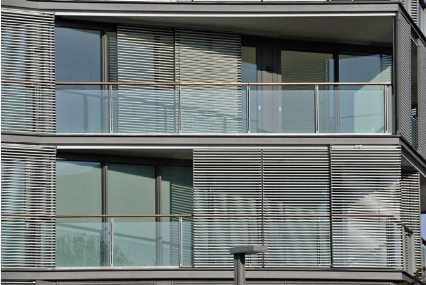
Fig. 1.18 Carlos Ferrater, Aquileia Tower , Jesolo. Diaphragmatic conception of the envelope according to the technical hybridization between transparent enclosures and external sunshade curtain textures. © Courtesy of Schüco
