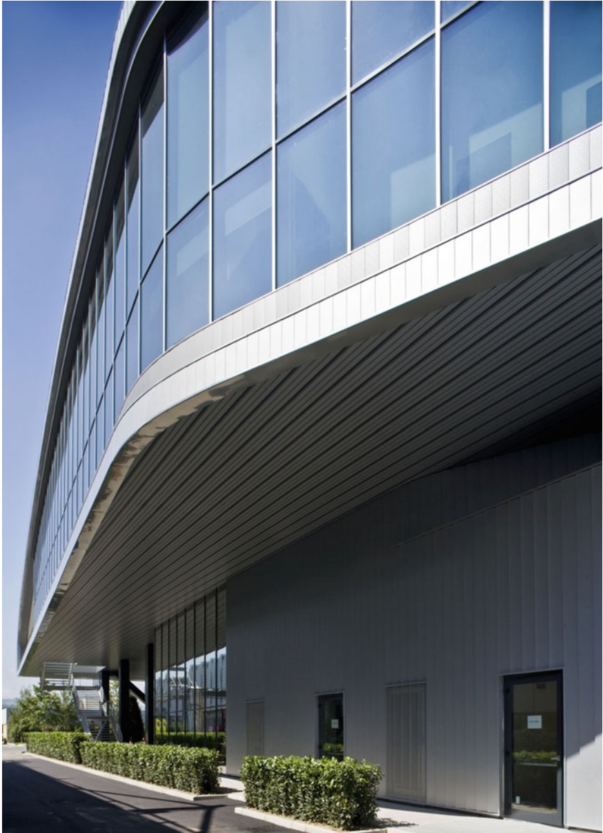
Fig. 1.2 MDN Marco Visconti & Partners, Ferrari Restaurant, Maranello (Modena). Articulation for double-glazed façade components inserted beyond the stringcourse banding marked by the stainless steel sheet metal casing (externally pronounced) and, in the upper part, by Rheinzink vertical slat cladding. © Courtesy of Wicona
